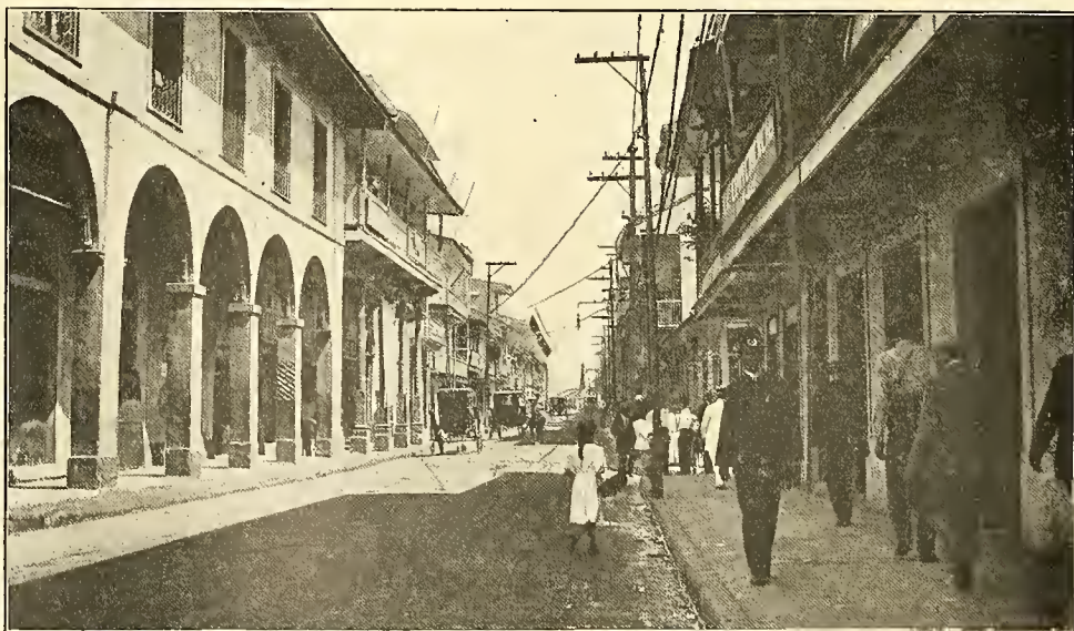
A STREET AFTER PAVING
